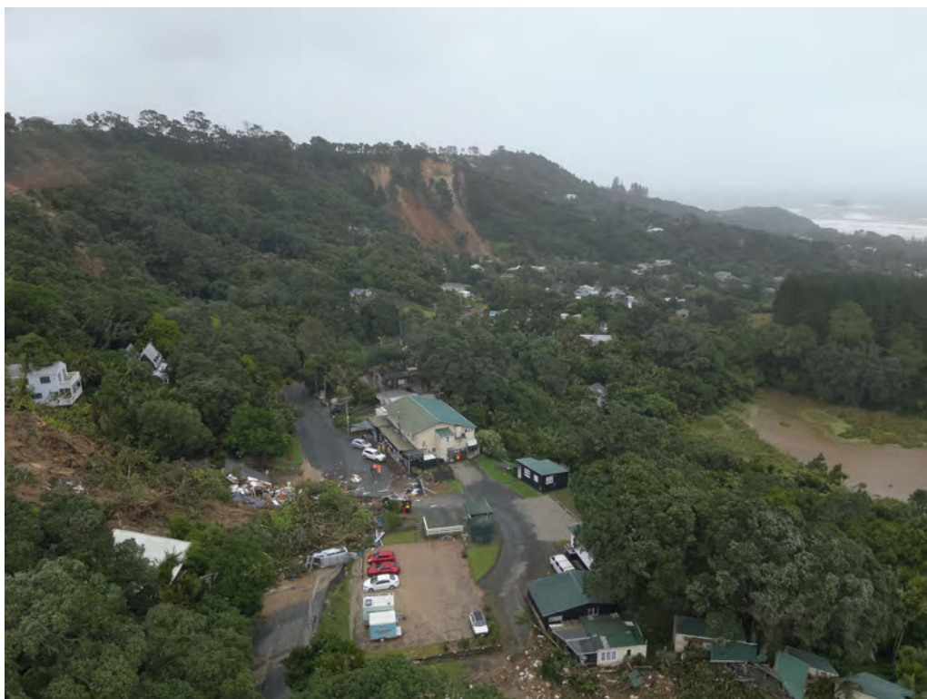
Figure 2 above. Rescue site in foreground where debris covers road. Lodge café is the large building in the centre past the rescue site. (USAR photo taken 14:00 hrs on 14 Feb)
