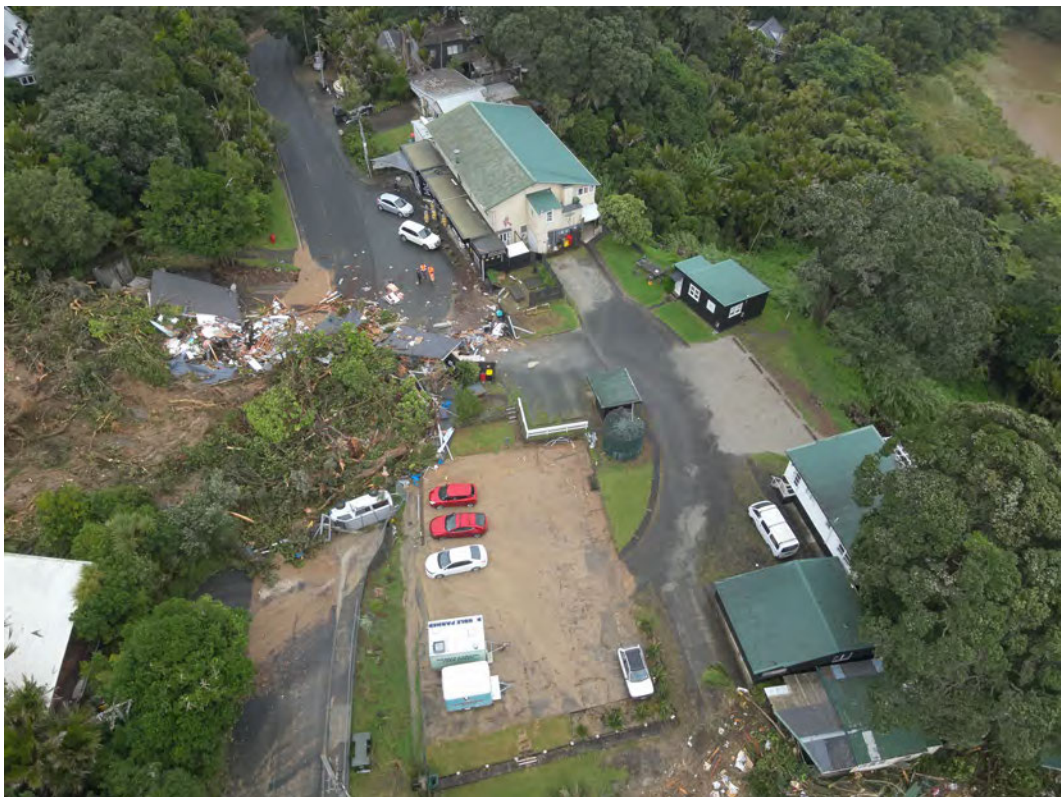
Figure 4 above. Close up of rescue site on roadway. (USAR photo taken 14:00 hrs on 14 Feb)
